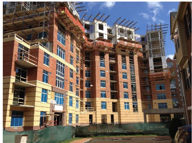
Figure 4: Site Photo of Swing Stage
